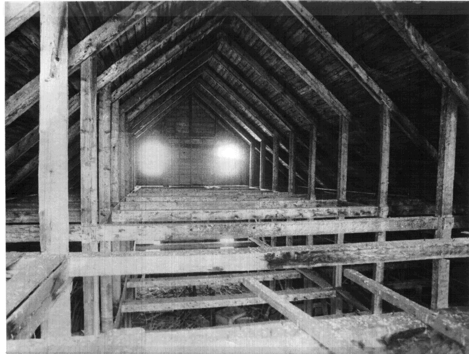
FIGURE 6: "B.B." WAREHOUSE, ATTIC
